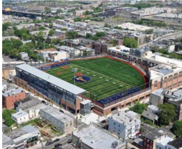
The rooftop athletic facility at the new high school in Union City, NJ, creates energy efficiency and saves space in a densely populated area. - COURTESY OF RSC ARCHITECTS
